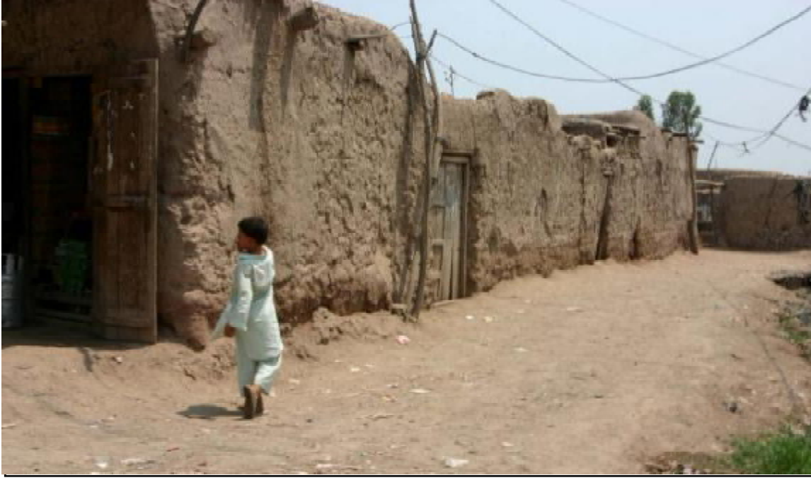
Many poor people live in mud-brick homes that have to be restored yearly.
